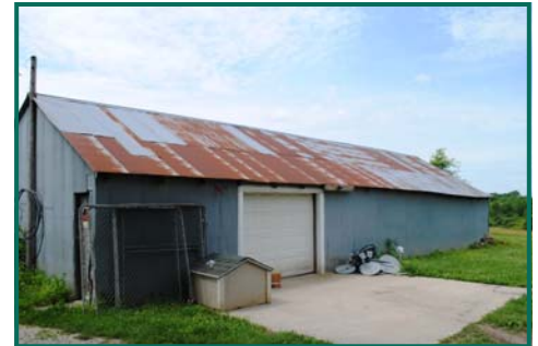
Parcel 2 - Machine Shed (Overhead Door)
