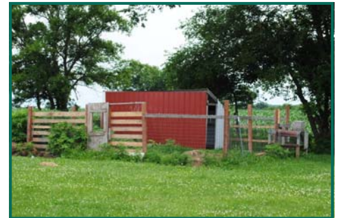
Parcel 2- Livestock Shed
